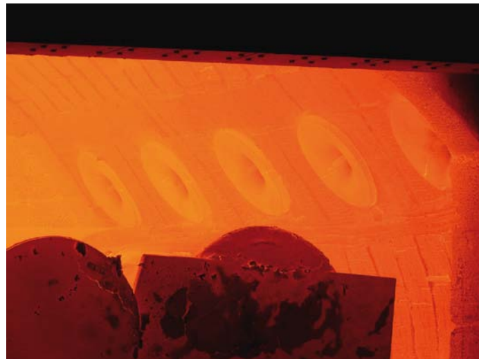
Fig. 4: flat flame burner in a bogie hearth furnace
